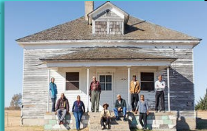
A group of descendants of the original settlers on the porch of one of the remaining historic buildings in Nicodemus.
